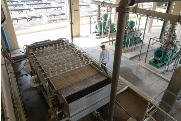
Chuck Redmond, PMP Plant Supervisor in the Sludge Thickening & Dewatering Building
